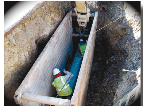
One of four temporary flow relief structures that will divert storm water flow to Lake Erie instead of back into area residents' basements.
