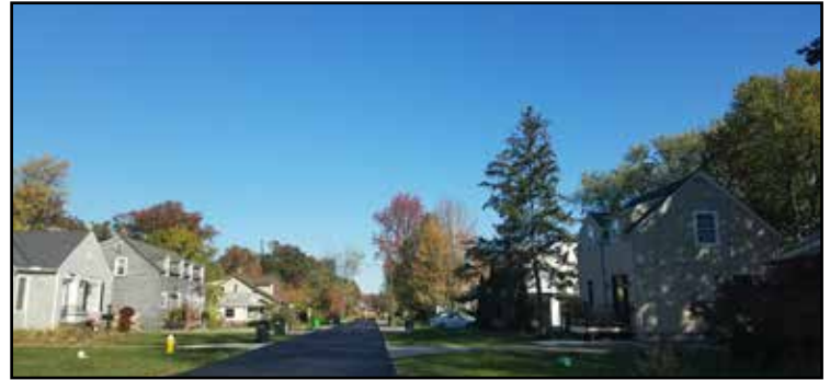
Stop 45 Area Combined Sewer Separation Project Restoration
