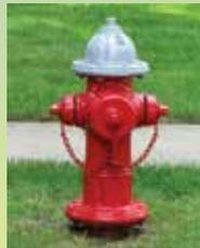
**FIRE HYDRANTS ARE DIRECTLY CONNECTED TO WATER LINES. IT IS OUR JOB TO BUY AND CONNECT FIRE HYDRANTS FOR EACH NEW WATER LINE AS IT IS BUILT.**
