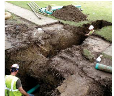
Typical sewer lateral construction
